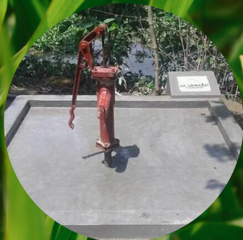
Completed hand water pump
